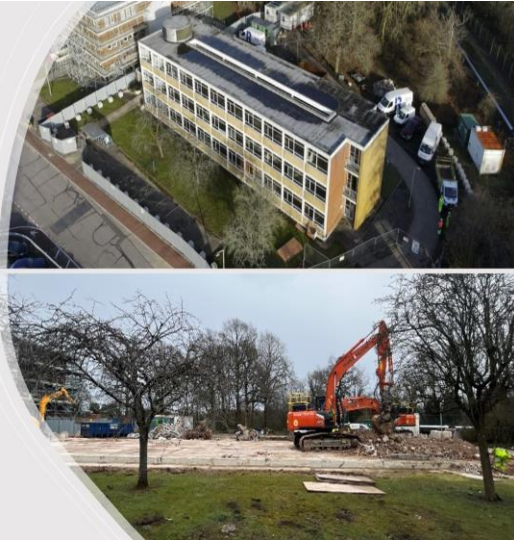
C21.1 Demolition Before & After
